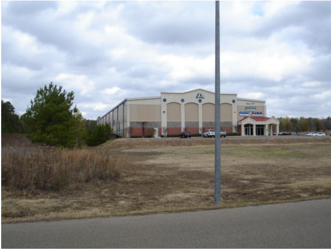
Figure 3: Looking north from the west boundary of Ward II Industrial Park toward the first tenant in the park, Allen's Electric Motor Service.
