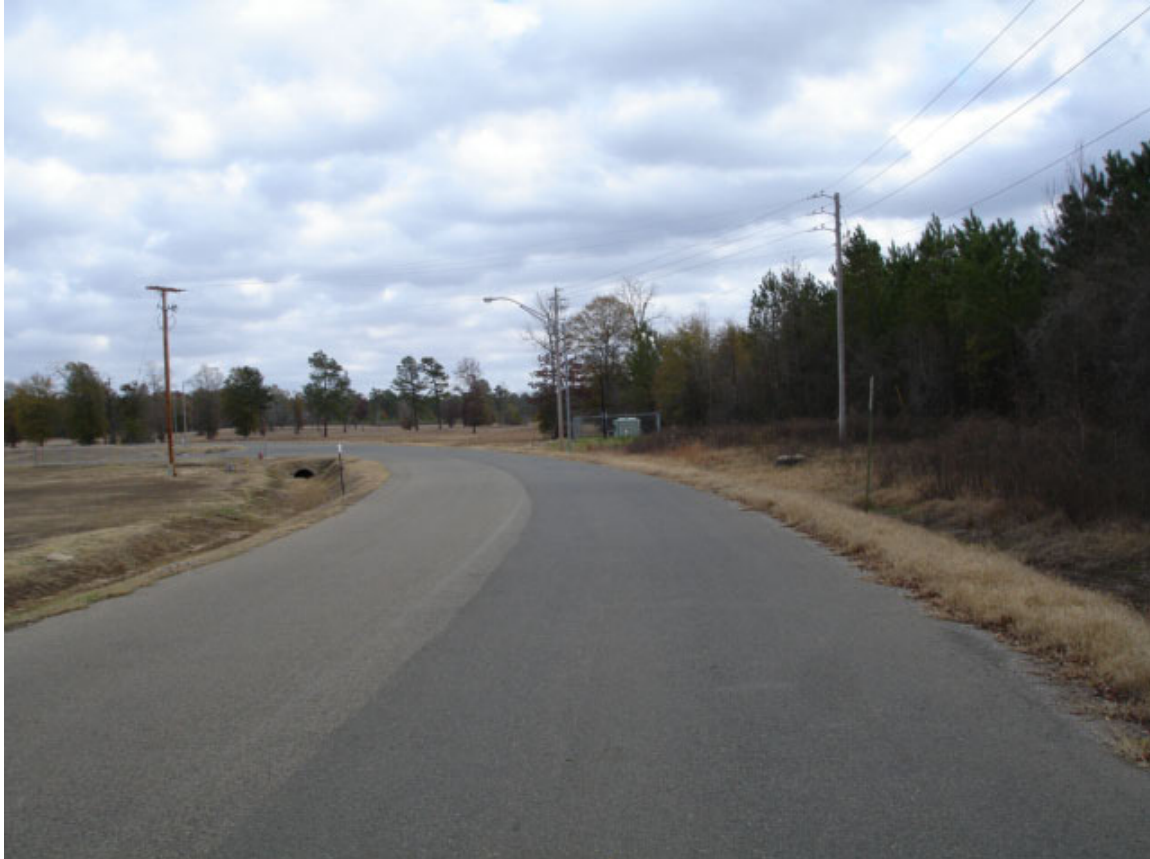
Figure 2: Looking east along Roy "Hoppy" Hopkins Drive at west boundary of Ward II Industrial Park with partially cleared property and a sanitary sewer lift station in the distance.
