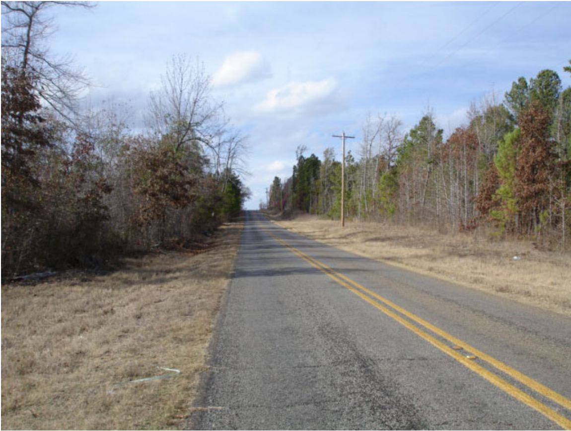
Figure 13: Looking north along LA Highway 170 from its intersection point with the future extension of Roy “Hoppy” Hopkins Road.
