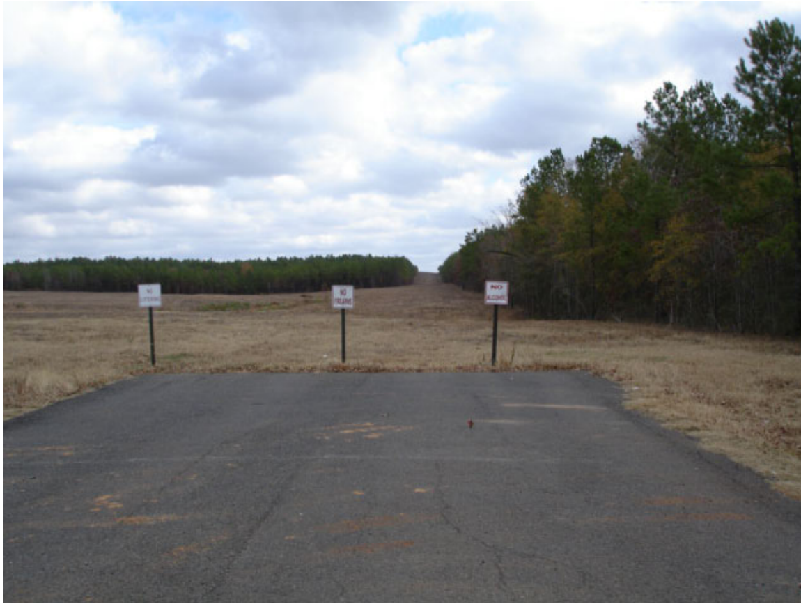
Figure 9: Looking east from the end of the paved portion of Roy “Hoppy” Hopkins Drive with the cleared right-of-way for the future roadway extension in the distance.
